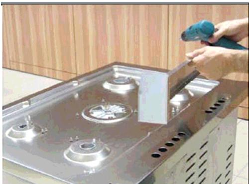
If the holes are not aligned, partially loosen the brackets at the back of the worktop as shown below.
