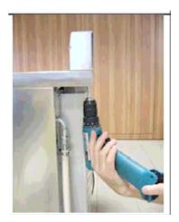
Position the back part of the backguard and secure it to the worktop tightening 4 screws from the bottom.
