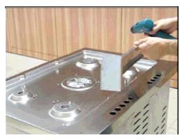
If the holes are not aligned, partially loosen the brackets att the back of the worktop as shown below.
