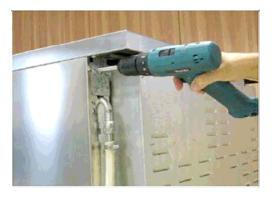
Install the front part of the backguard by tightening the 2 central screws from the top and
