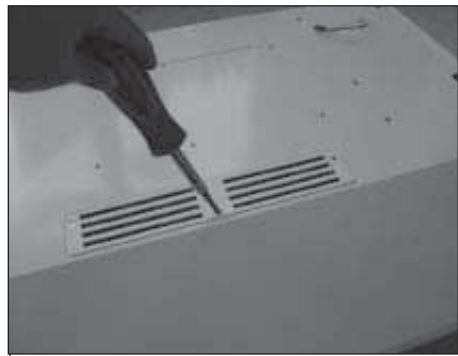
7. Place louvered recirculating plate over top opening and secure using the screws previously removed.
