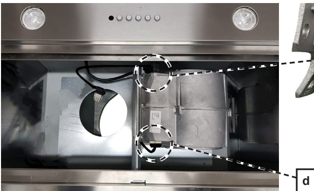
Detail of the first blower.
