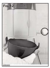
Utility valve (circled in **Fig. 12**), next to power unit, can be used to service area around where power unit is installed.
