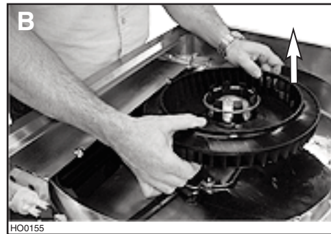
Lift the blower wheel to remove and set aside.
