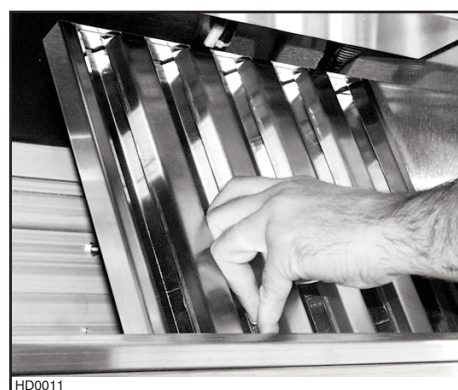
BAFFLE FILTER (TYPICAL)
