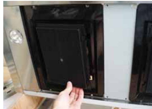
3. Install charcoal filters into charcoal filter brackets
